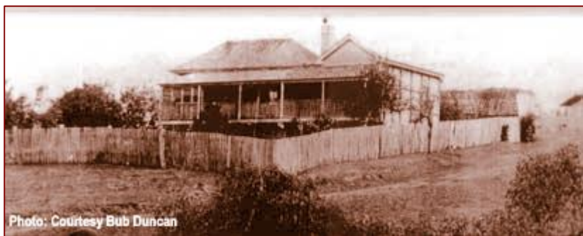
Quarantine Keeper's Residence
